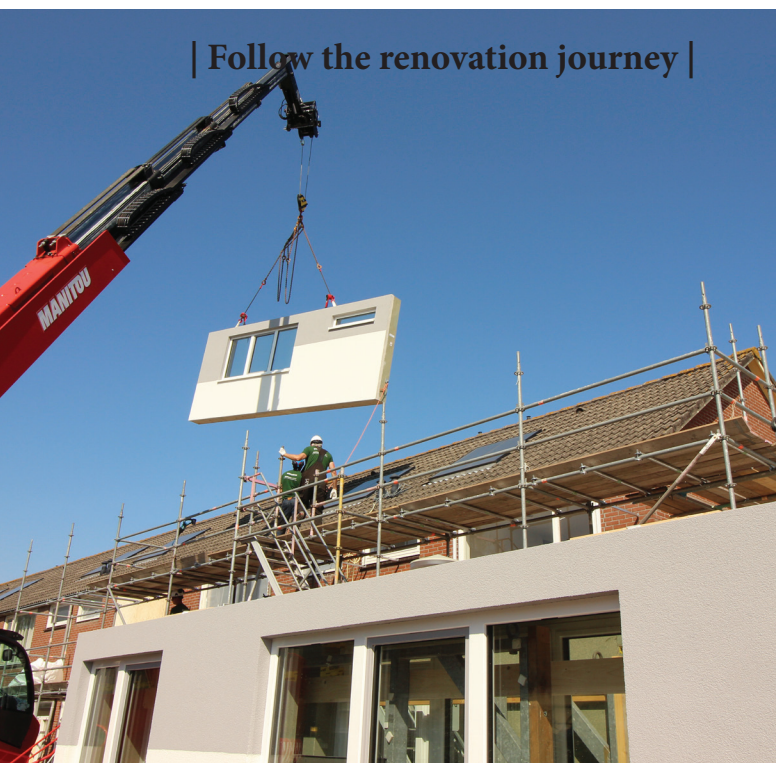
Pre-fab panel mounting | © Chris van den Bos, Van Dillen Bouwgroep - Pre-fab window and doors production & before
